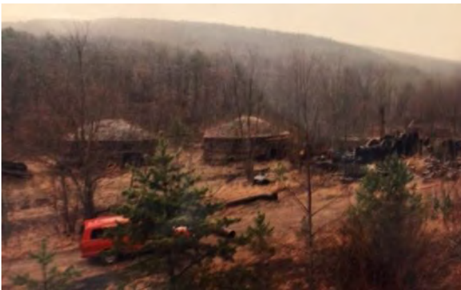
Several ovens in the Brickyard
