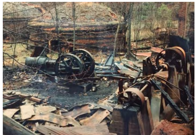
Engine and other machinery
