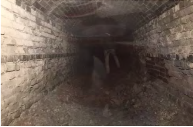
James Wilson exploring the underground ductwork
